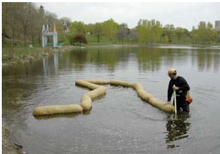
A barley straw installation project helps control algae in Powderhorn Lake.
