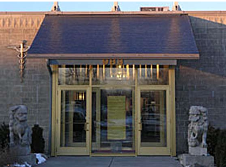
This retrofit, incorporating solar shingles into the design of a Minneapolis business, demonstrates how solar energy can be both practical and visually appealing.
