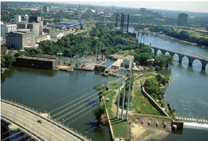
Saint Anthony Falls in downtown provides enough clean electricity for approximately 13,200 homes annually through a hydropower plant operated by Xcel Energy.
